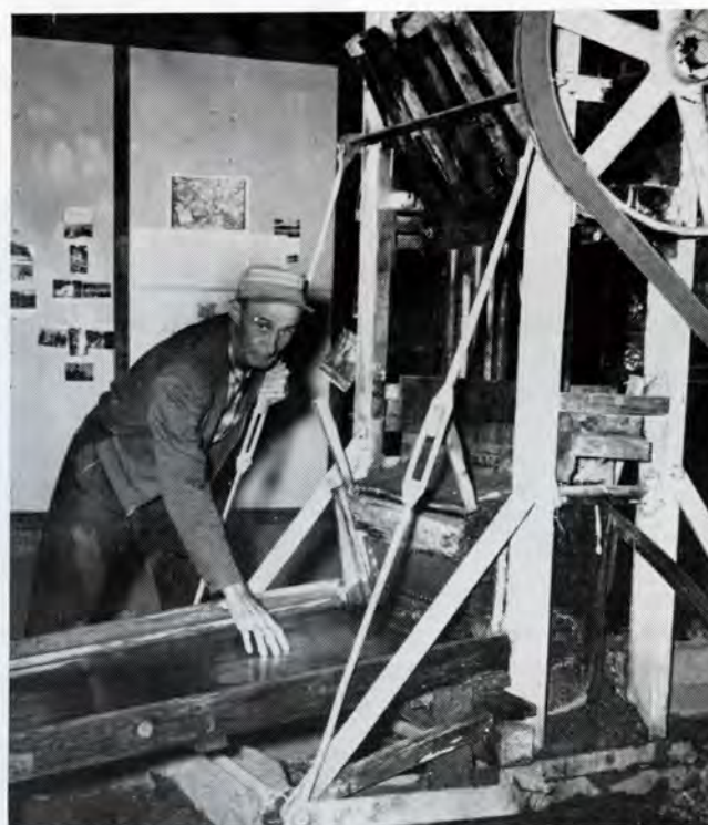
THIS small stamp mill was used for testing small batches of ore and is still operated at Dahlonega Gold Museum
