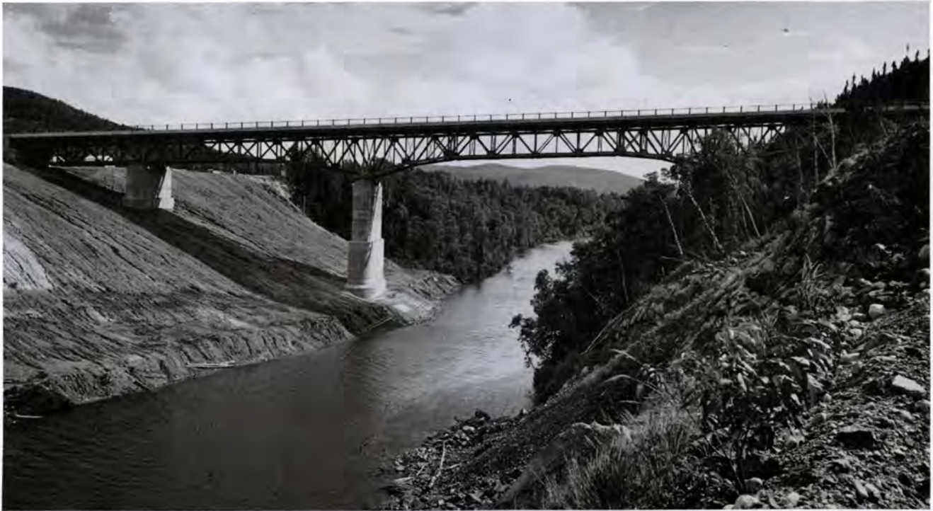
BRIDGE over Little Pic River along the Trans-Canada Highway
