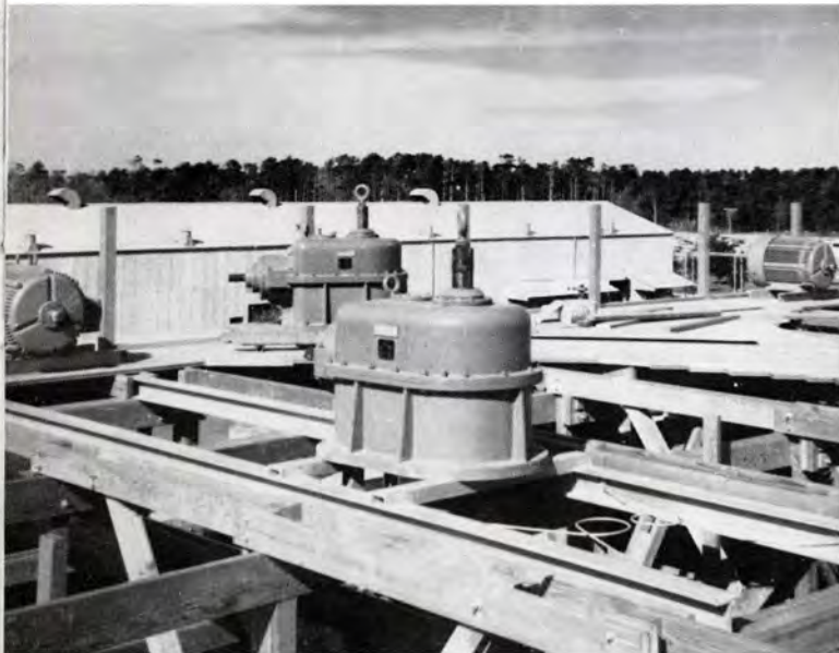
TWO LUFKIN Model DVB-80 Double Reduction Gears operating for Continental Oil Company. Tower is located at Lake Charles, Louisiana, and was built by Slough-De Flon Company. Rating of gears: 100 HP at 10.7 to 1 ratio, 1750 RPM input
