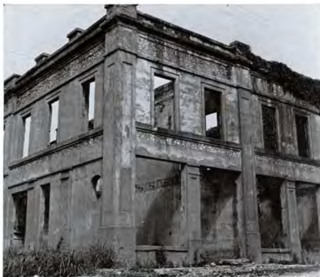
RUINS of the bank at Monte Ne
