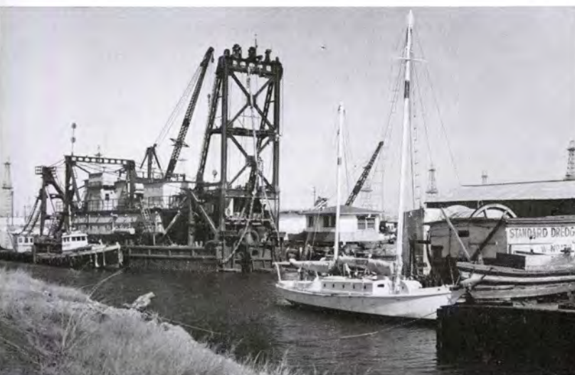
STANDARD Dredging Co. of Wilmington, Calif. owns Harbor Dredge "Los Angeles" for hoist duty, using a Lufkin Model D340 reduction gear rated at 200 HP
