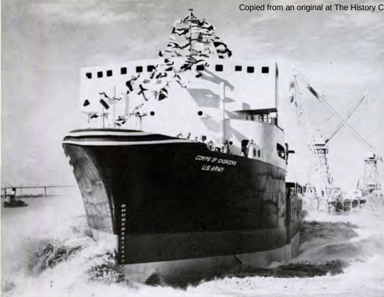
IN JUNE, 1959, Hopper Dredge Markham was launched equipped with two Lufkin Model C8414 compound gear reducers rated 2730 HP
