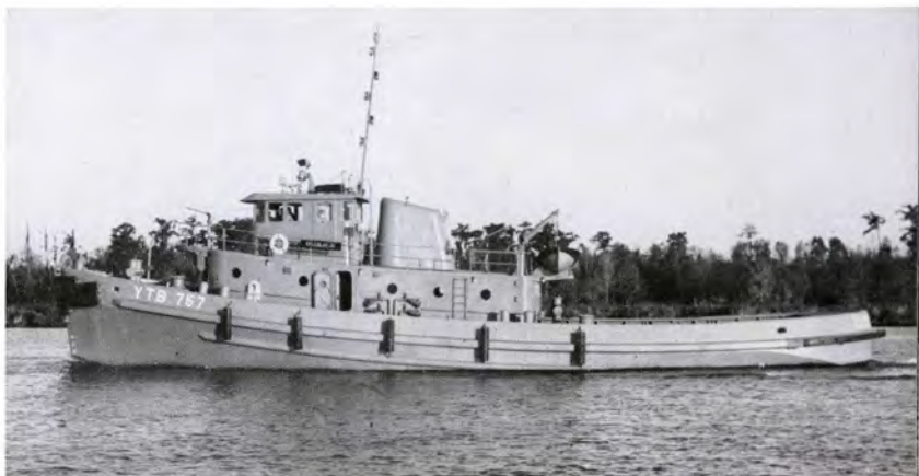
NAVY Harbor Tug YTB "Oshkosh" is propelled by a Lufkin Model RS4222 reverse-reduction gear, 2000 HP
