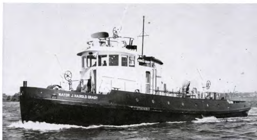
BALTIMORE Fireboat "Mayor J. Harold Grady" uses a Lufkin Model V1614 reduction gear, rated 880 HP
