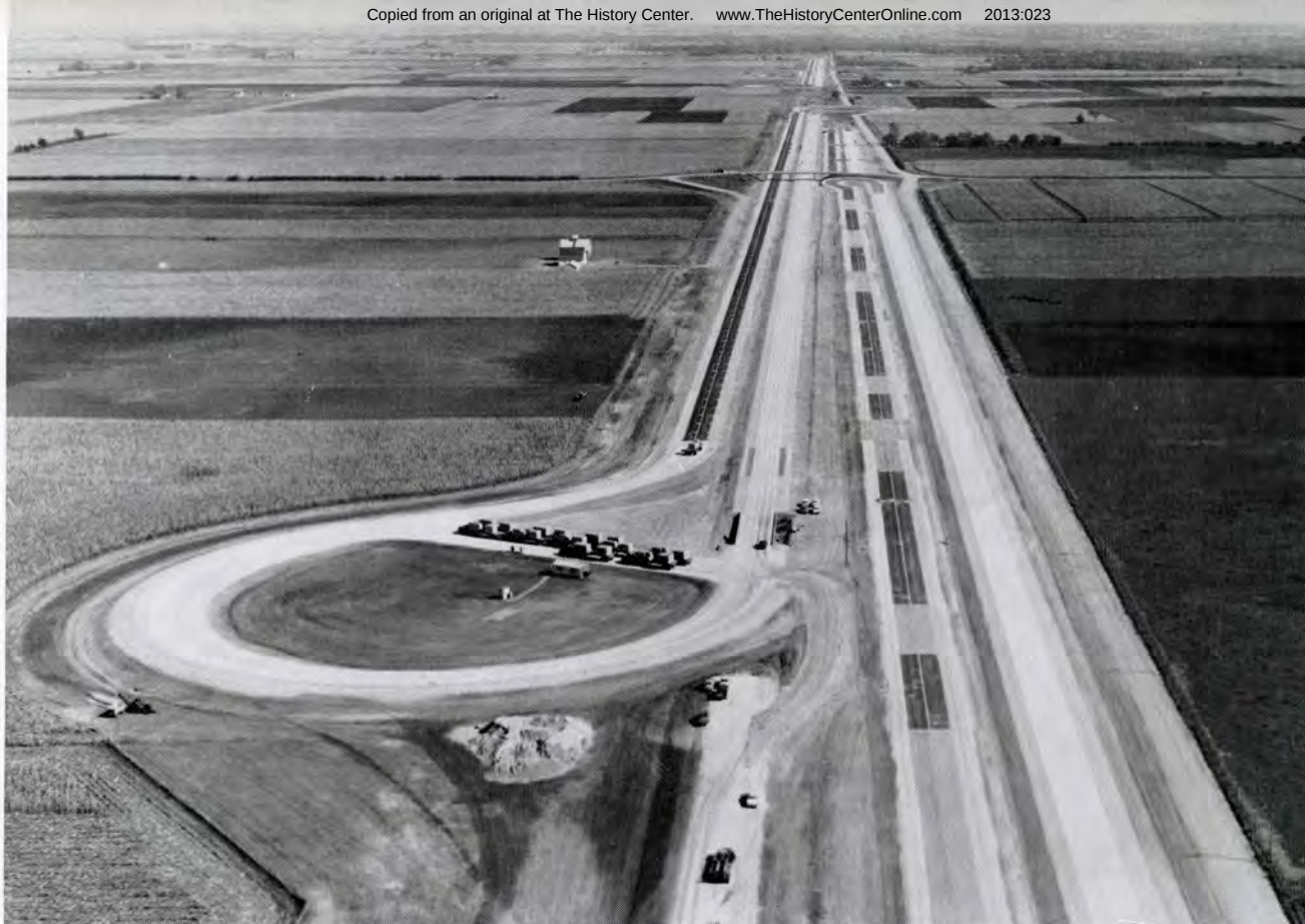
THIS aerial view shows about one-half of the test pavement. Four large test loops, like the one at left, were built end-to-end along an 8-mile stretch
