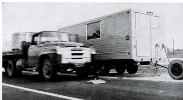
MEASUREMENTS of transient effects of load on test pavements are recorded by relatively complex electronic equipment installed in movable vans
