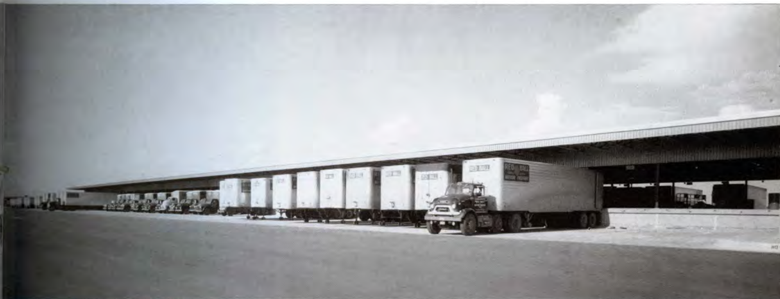
RED Ball's new 500-foot dock facilitates the movement of more than five million pounds of freight daily
