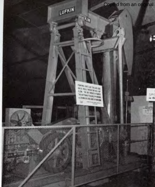
THIS Lufkin A-160D-74-25 Air Balanced Pumping Unit, driven by a Lufkin HC-333B Engine was on display at the stockholders meeting of the Standard Oil Company held at Lawrenceville, New Jersey.
