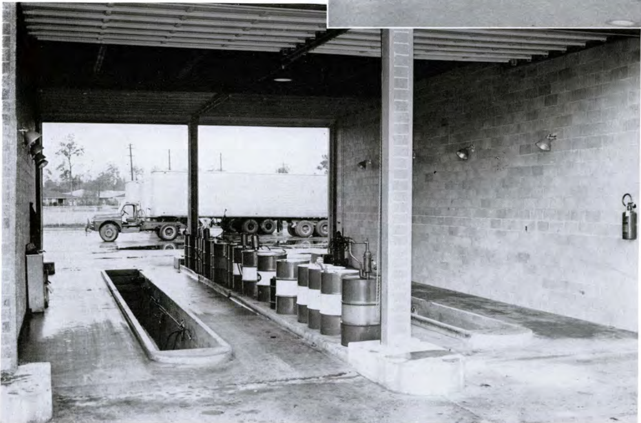
THESE two grease pits house modern lubrication equipment to keep Red Ball's fleet in peak condition
