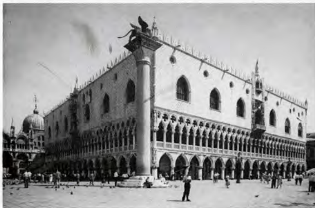
DOGES' Palace contains glorious state apartments filled with paintings and rich ceiling frescoes
