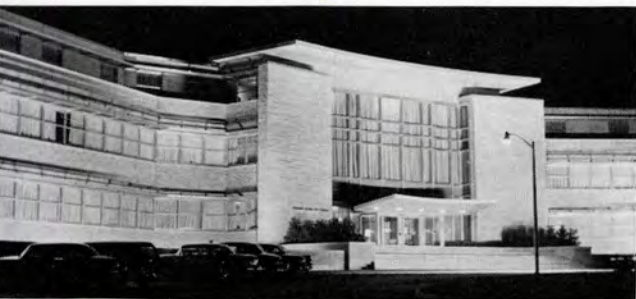
New Office Building of STANDARD-VACUUM Oil Company located at 1000 Westchester Avenue, White Plains, New York. The new offices house the overseas operations of this company which serves 50 countries and territories in Asia, Africa and Australia
