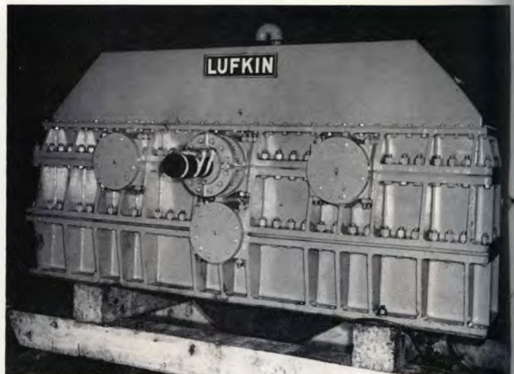
THIS is largest gear drive ever built by Lufkin; it's twice as big as largest pumping unit gear.
