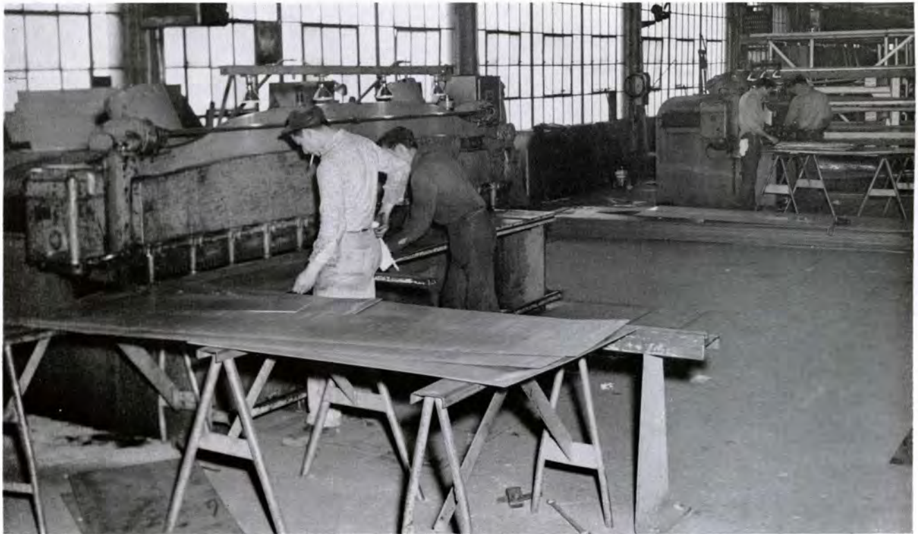
1 THE flow of material starts at the shearing machine where blank sheets are cut to specified sizes
