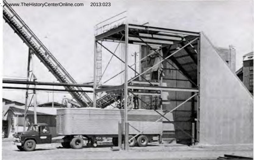
HERE , chip-hauling trailer is backed up to a hopper at a paper mill, in position to dump its load of chips
