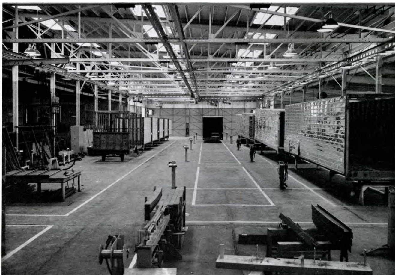
8 ASSEMBLY line of new van shop has work stations with electrical, gas, air, oxygen and water
