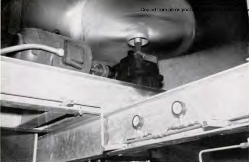
FORTY Lufkin right angle type VB gears operate aerial coolers in Signal's Tioga gasoline plant
