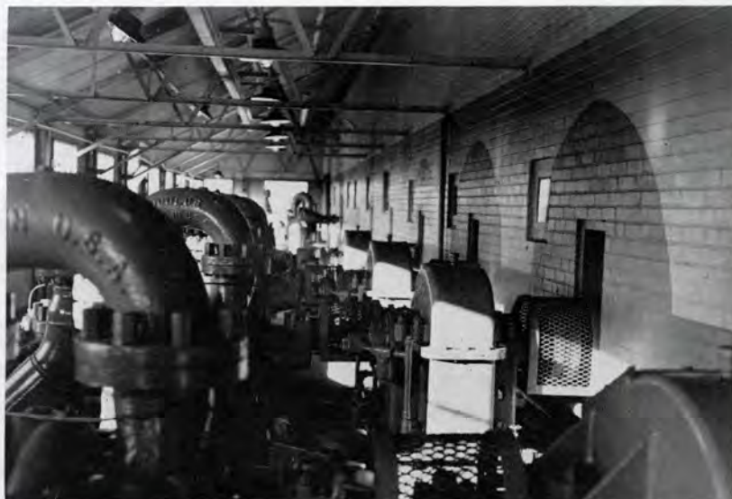
VIEW of pump room at Gaines Station showing gear increasers equipped with Lufkin herringbone gears
