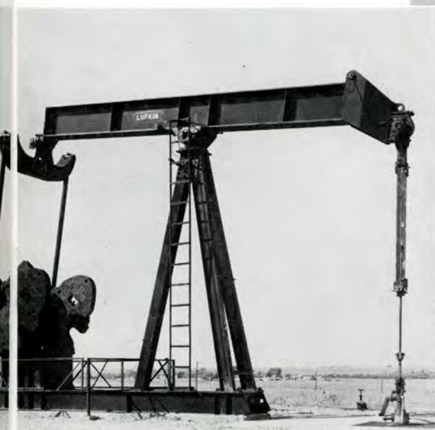
LUFKIN TC-1A-54B Pumping Unit in North Burbank Field, Osage County, Oklahoma
