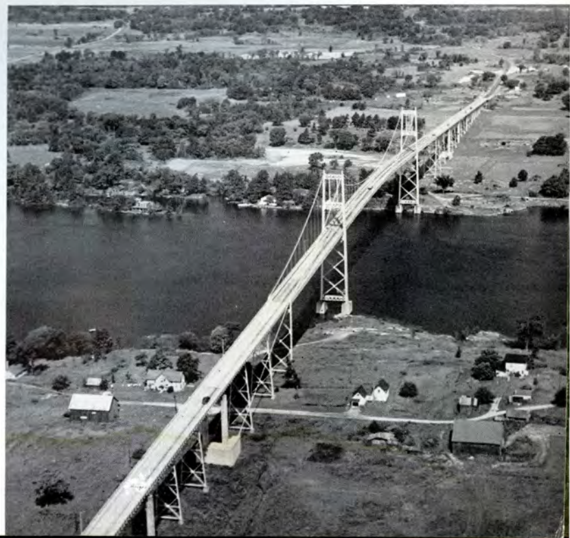
THE AMERICAN span of the Thousand Islands bridge links U. S. shore at Collins Landing with Wellesley Island
