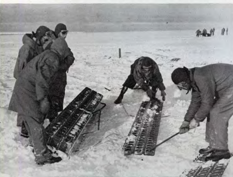
WEARING special sun glasses to protect eyes from snow glare, these men lay an airstrip on the ice
