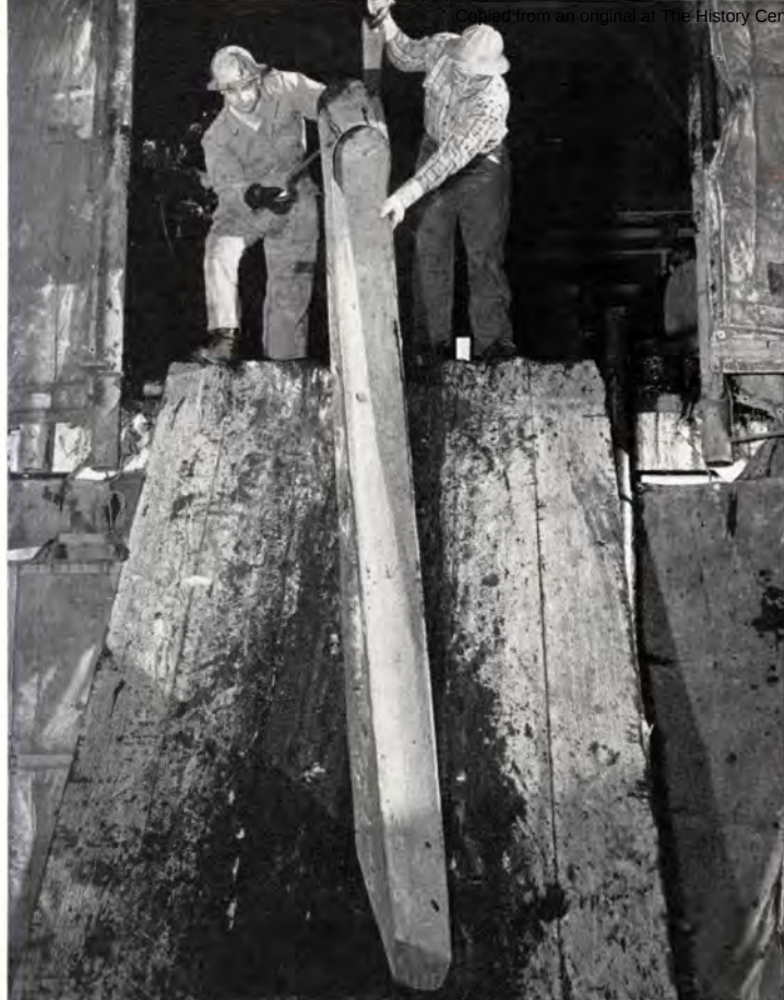
Above: Designed by engineers for directional drilling, the Whipstock was so named because it resembles the dashboard receptacle on which buggy whips were once kept by oil men. Made of a cylindrical steel casting, it has an inclined groove so drilling bit can turn off vertical course.
