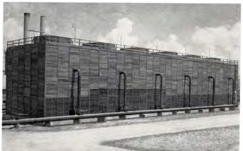
Designed and constructed for a large Texas oil refinery, this is the modern six-cell mechanical draft cooling tower.
