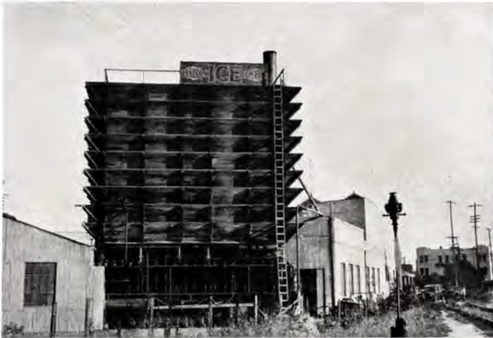
This atmospheric cooling tower was built in early 1900 by Santa Fe Tank and Tower Company. Despite its antiquity, it remains in service today and is doing its work.
