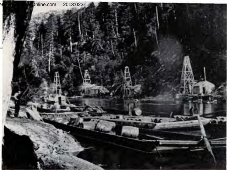
Transportation, in the early days of oil, was a tough problem. The first carriers were flat bottom barges used to float the barrels of oil down stream. The oil industry now uses railroad and truck tanks, barges, pipelines and sea-going tankers to move its products.
