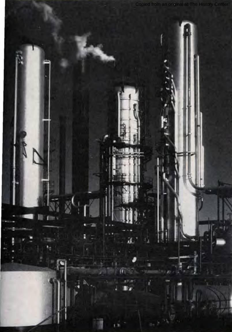
This crude section of a leading oil company's refinery is part of a gigantic network of refineries which covers the land across America from coast to coast.
