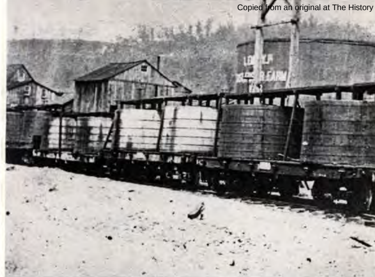
The first railroad tank cars were put in service in 1865. They were merely two huge wooden tanks or vats mounted on a flat car, holding 40 to 50 barrels of crude oil. Today's tank car holds 10,000 gallons.
