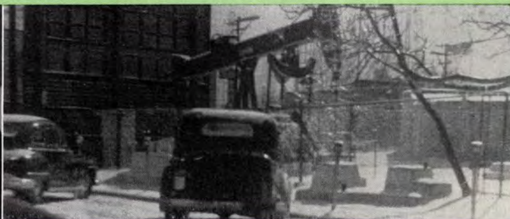
This picture was taken in Kilgore, Texas, after the February snow storm. It shows a LUFKIN unit with horsehead on each end of the walking beam. The unit is pumping two wells simultaneously. There are three such double end walking beam set-ups in a row on this street in downtown Kilgore.
