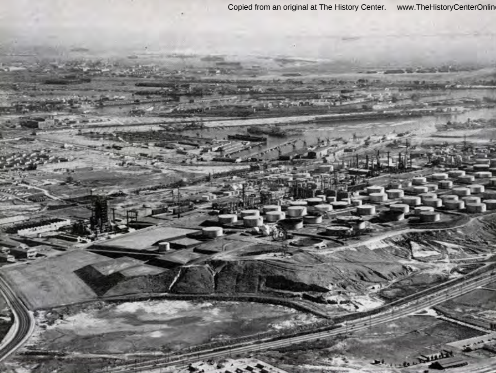
AN AERIAL VIEW of the Los Angeles refinery of Union Oil Company. This is one of four modern plants operated by this pioneer, western petroleum organization. Last year the Company processed 43,000,000 barrels.
