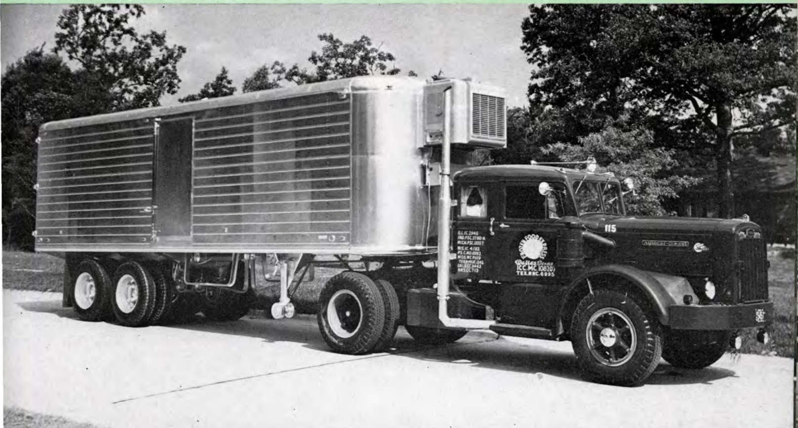
Below: LUFKIN'S NEWEST BABY is this aluminum refrigerated van considered to be the lightest on the market today. It is used to transport such commodities as fish, shrimp and beef halves which require a temperature of zero or less. Also frozen fresh foods are hauled in these vans.
