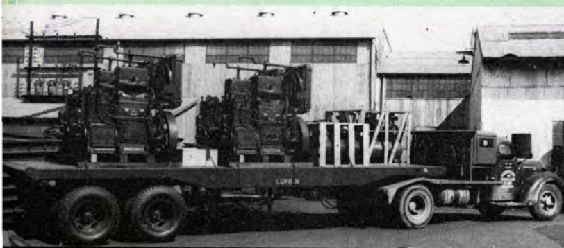
LUFKIN TRAILER PLANT has been building this tandem, self-loading standard oil field float longer than any other type trailer. Because of its primary interest in the oil industry, Lufkin perfected a float for moving oil field equipment or machinery.
