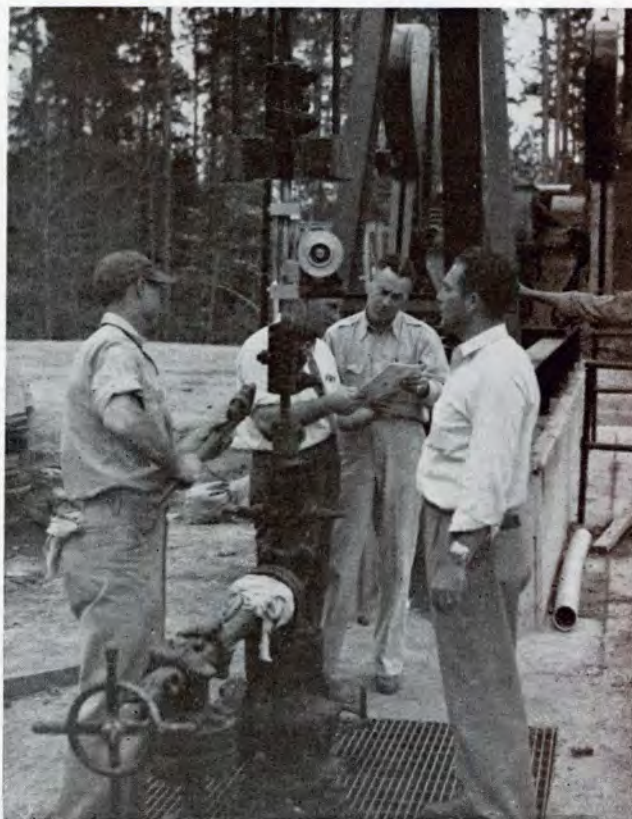
USING DYNAGRAPH to weigh 10,441-foot string of rods on pumping installation in Brookhaven, Mississippi, Field.
