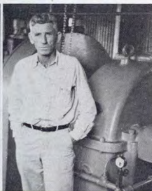
J. E. GALLIMORE Southern Pipe Line Co., Agua Dulce, Texas
