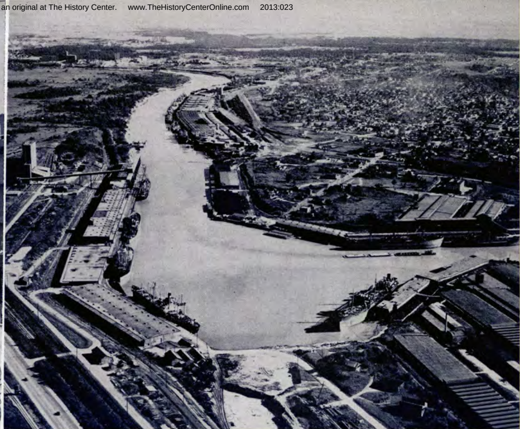
AERIAL VIEW of the Turning Basin of the 34-foot deep Houston Ship Channel, which extends for 50 miles across the Texas coastal prairie before entering the open waters of the Gulf of Mexico.
