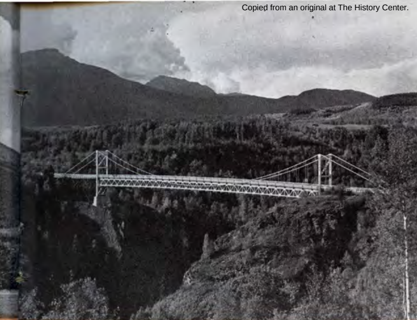
Hagwilget suspension bridge over the Bulkley canyon near Old Hazelton. Recently built, this modern span replaces a crude suspension bridge built by Indians many years ago from materials abandoned by the Western Union Telegraph Company's ill-fated Overland Telegraph project, which was to connect Canada with Europe through Siberia. Completion of the first Atlantic cable in 1866 stopped all work on the line.
