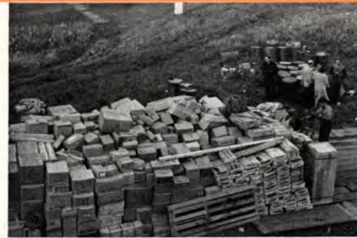
Here the pre-fabricated houses were unloaded for coal miner W. W. Wrigley.
