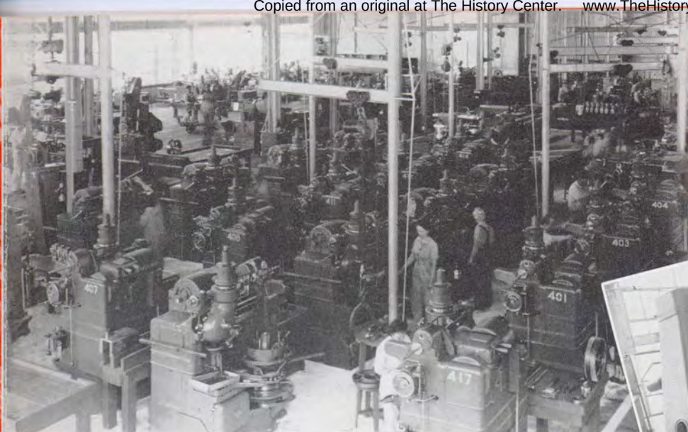
Above: Some idea of Lufkin's gear cutting facilities
