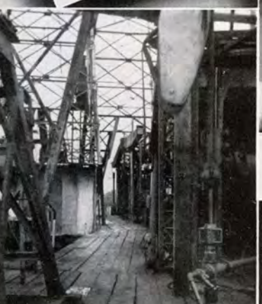
Five wells on one floor—one of the smallest leases in the world, 60' by 140'. Four walking beams shown in picture. Santa Fe Springs, Cal.
