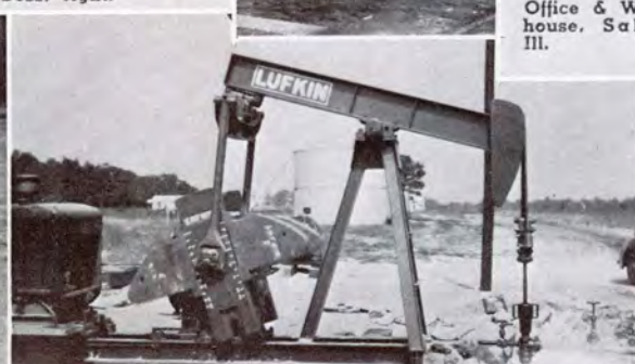
Lufkin TC 77-3 Unit installation for Carter Oil Company, Dix field, Ill.
