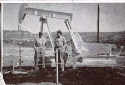
Lufkin TC 66-5A Unit Assembly; installation of the Basin Oil Properties, Inc., McCamey field. One of 5 such installations. Oliver Inman, Supt., left; Ernest Pendleton, Farm Boss, right.
