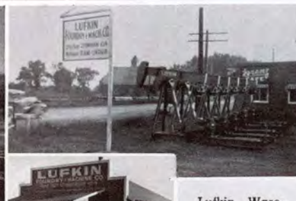
Lufkin Warehouse, St. Elmo, Ill.
