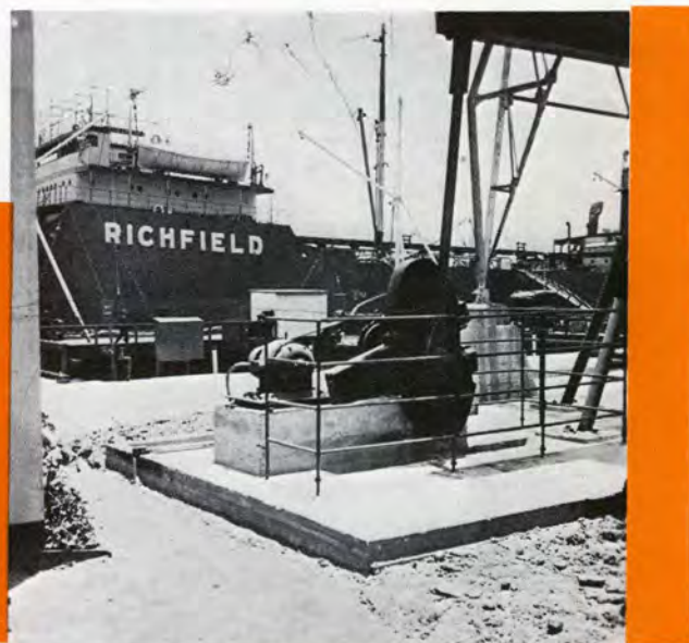
RICHFIELD OIL COMPANY'S LUFKIN INSTALLATION at the Wilmington harbor in their refinery area
