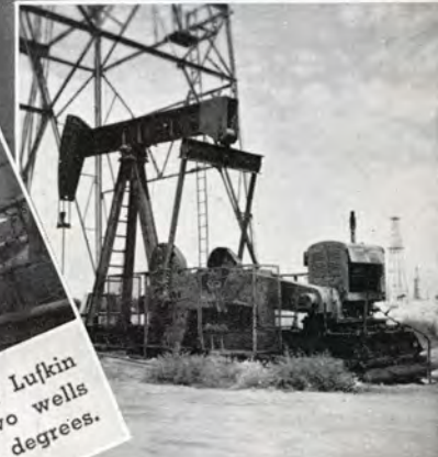
Shell's Mountain View installation of Lufkin T. C. 1-41 unit assembly.
