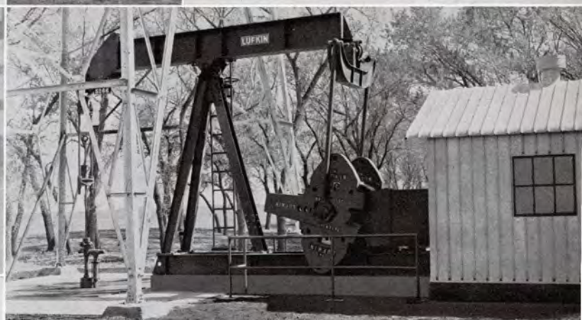
Atlantic Oil & Refining Co., Lufkin TC 2A-26 Unit Assembly, St. John, Kansas.
