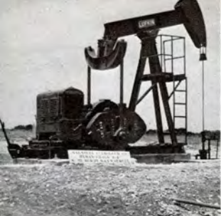
Lufkin installation for Magnolia in Mitchell County, West Texas.
