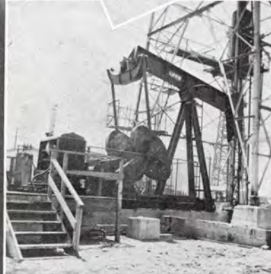
Texas Company, Foix No. 6, Santa Fe Springs. Installation is Lufkin T. C. 1-41 unit assembly.
