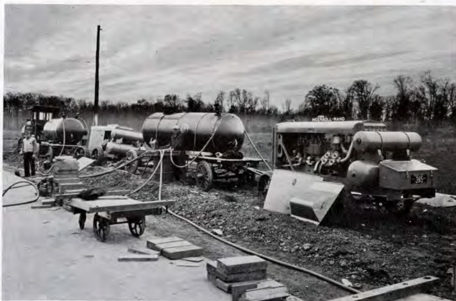
SOURCE OF AIR SUPPLY —Two 210-cfm., air-cooled, portable compressors are stationed midway of the strip being moved. To provide a large volume of air for instant use, each machine discharges at 100 pounds pressure into a 4 x 12-foot portable receiver. Two air lines run from each receiver to the hose being inflated, the air being fed simultaneously at four equidistant points.
