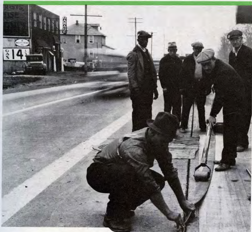
THE FIRST STEP —After the bituminous filling has been removed from the longitudinal expansion joint, a 3-inch linen fire hose is inserted in the crack, being rolled as shown to flatten it. By inflating this hose, the right-hand strip of pavement is pushed over until the opening is 2 inches wide. Subsequent moves are then made by successively inflating and deflating a 6-inch hose.
