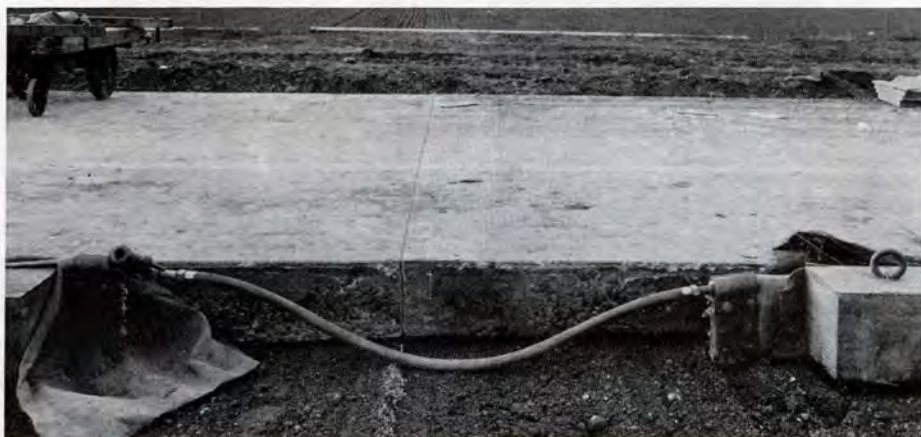
CONNECTION OF HOSE SECTIONS —The hose which is inflated is not continuous, there being a 27-foot length for each 35-foot slab of concrete. These sections, or "bags" as they are termed on the job, are connected by standard \frac{3}{4} -inch air hose. At the left may be seen one of the valves for exhausting the air after each shove.
