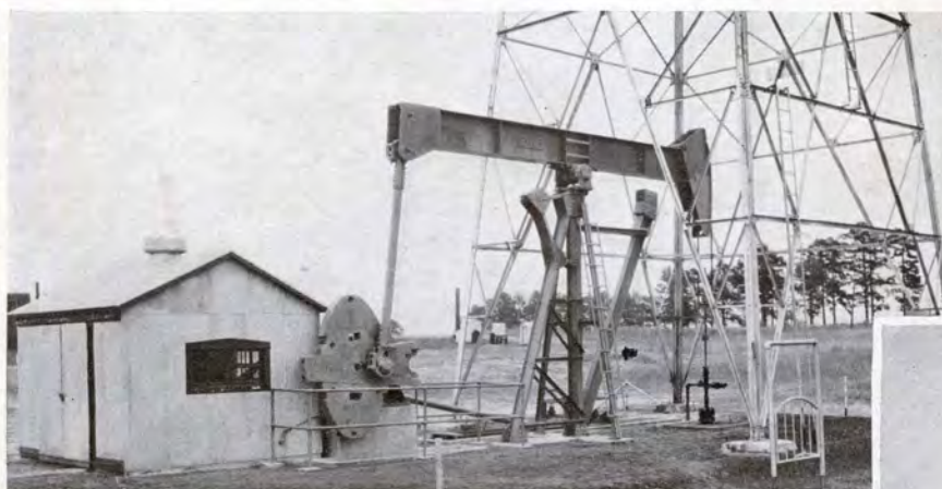
Lufkin single crank unit. Devonian Oil Company, East Texas.
