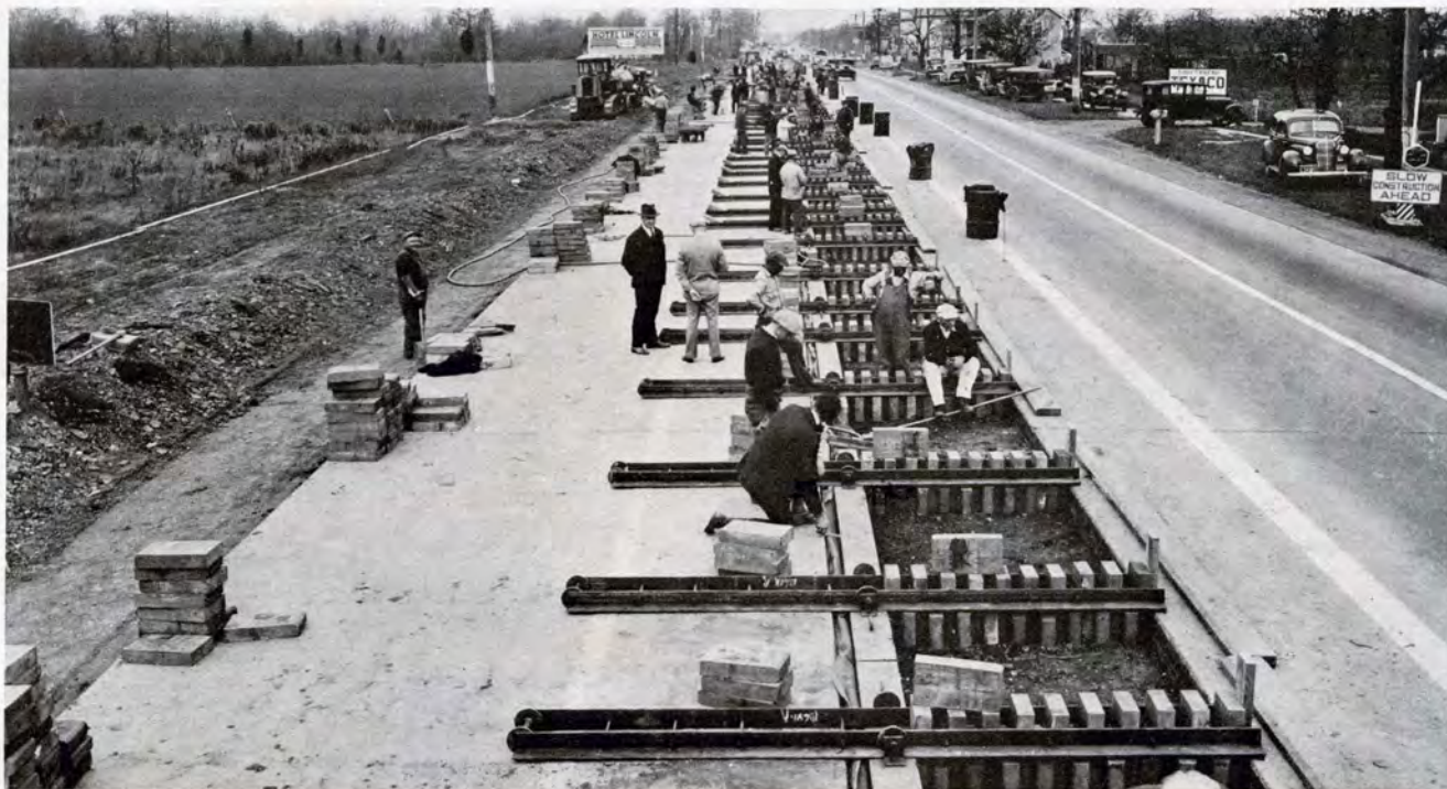
GENERAL VIEW OF OPERATIONS —This picture was taken during the moving of a strip of pavement 455 feet long and consisting of thirteen slabs each 14\frac{1}{2} \times 35 feet. It shows details of the apparatus developed to facilitate blocking-up behind the air hose after each move.
