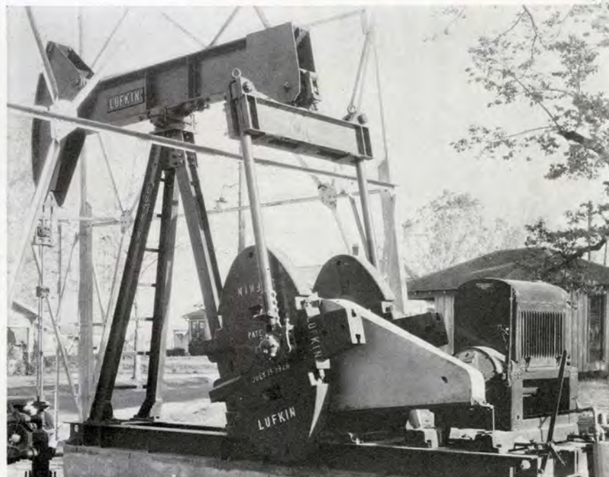
Lufkin Twin-Crank Unit—Phillips Petroleum Co. near Gladewater.—Photo by Ward, Tulsa.
