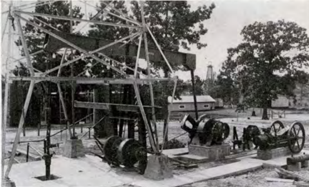
Lufkin No. 56 Heavy Duty Herringbone Unit with Center-line Beam Assembly and No. 6 Rod and Tubing Hoist—single cylinder engine drive. Woodley Petroleum Company, George Thompson No. 3. Twelve such installations for Woodley.
