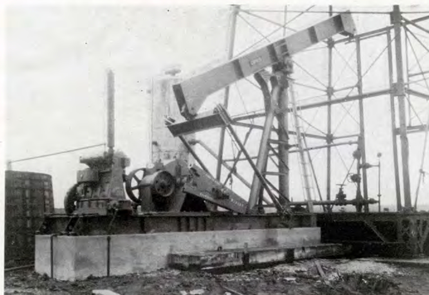
Recent Oklahoma City installation Lufkin No. T. C. 1-A-56-1028-C Unit. Note old foundation. After laying foundation for competitive unit this Lufkin was installed—a saving even though original foundation was lost.
