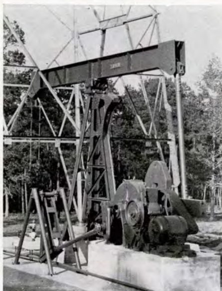
Lufkin Twin Crank Unit Assembly with structural base arranged for gas engine drive. Sinclair Prairie Oil Company, Laurther Lease.
