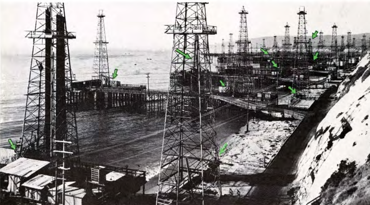
Ellwood Field, Goleta, California—mountain-side view. Thirty-one Lufkin Units are now in operation in this field—a few visible as indicated by arrows.
