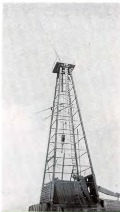
CROWN BLOCK PROVIDES NEAT HIDING PLACE FOR LOST TOOLS —Unretouched photo of what happened when tools blew out of hole. After exhaustive search tools were finally located hanging from crown block as will be seen in photo. I.T.I.O.-Barnsdall well, Rogers lease, Okfuskee County, Oklahoma.—Photo courtesy C. O. Rison, Division Supt., I.T.I.O. Mr. Rison was in charge of drilling this particular well.
