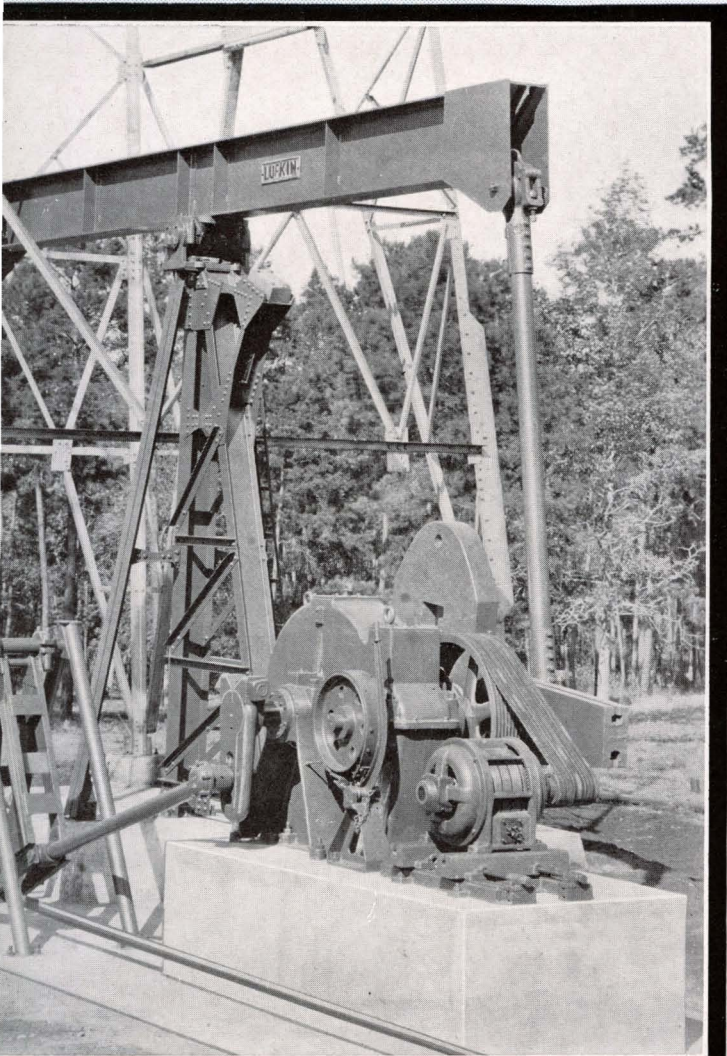
Close-up of Leschner & Hubbard installation in the Castleberry survey. Equipment includes Lufkin No. 58 H.B. Unit with "Back-side" crank with underslung swing take-off and Lufkin center-line Post-Beam-Pitman assembly, General Electric motor drive
