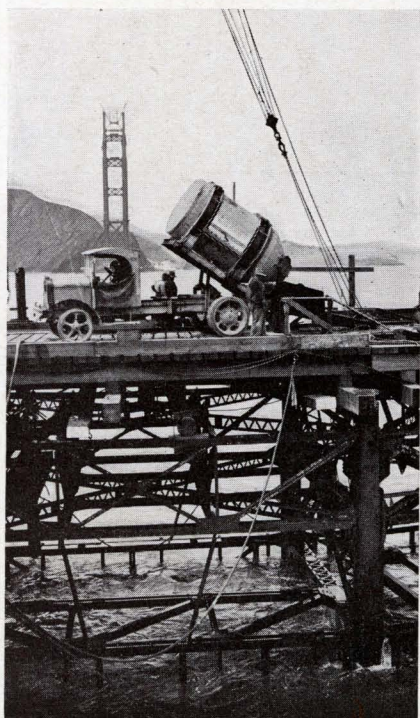
Showing method of pouring premix concrete—south pier and fender wall construction, San Francisco side. In the background 4200 feet across the waters of the Golden Gate to the north can be seen, the Marin Tower construction.
