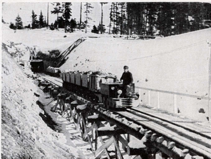
View at West Portal, showing a rock train on its way to the dumping ground. Driving a tunnel through the Continental Divide means moving plenty of rock to make room for water.
