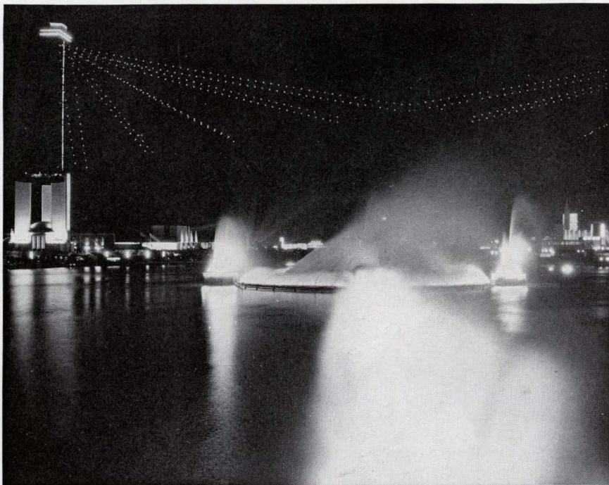
NIGHT SCENE AT "A CENTURY OF PROGRESS"—Federal Building, electrical group and the east tower of the Sky Ride as they look at night. The Sky Ride towers and cables are brightly illuminated for the first time this year. Gleaming and bright is the World's Fair for 1934.
