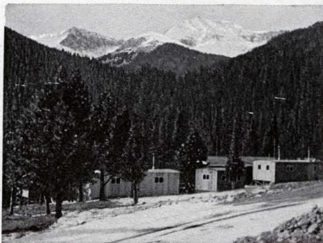
Below—The workmen's camp occupies a scenic spot near the east portal of the tunnel. Center—Mr. Platt Rogers, Jr., president and general manager of the contracting firm.
