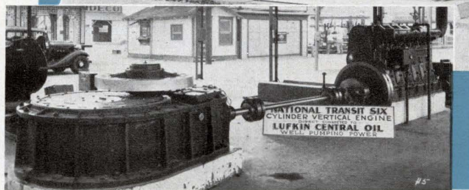
Lufkin No. 150 Herringbone power driven by National Transit Six-Cylinder Vertical engine.
