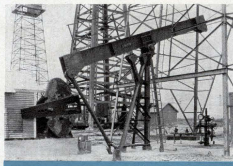
Sun Oil Company Wilbur No. 15, Barbers Hill: This Lufkin Unit and other Lufkin equipment is all set to go when the well stops flowing.
