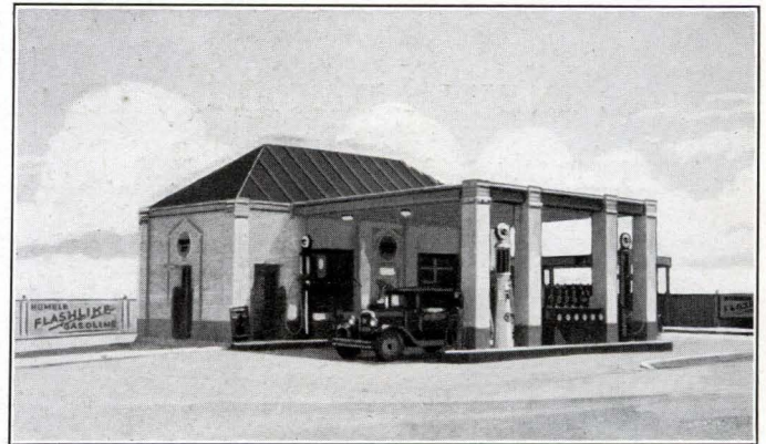
Type of service stations erected in Lufkin by the Humble Oil & Refining Company.
