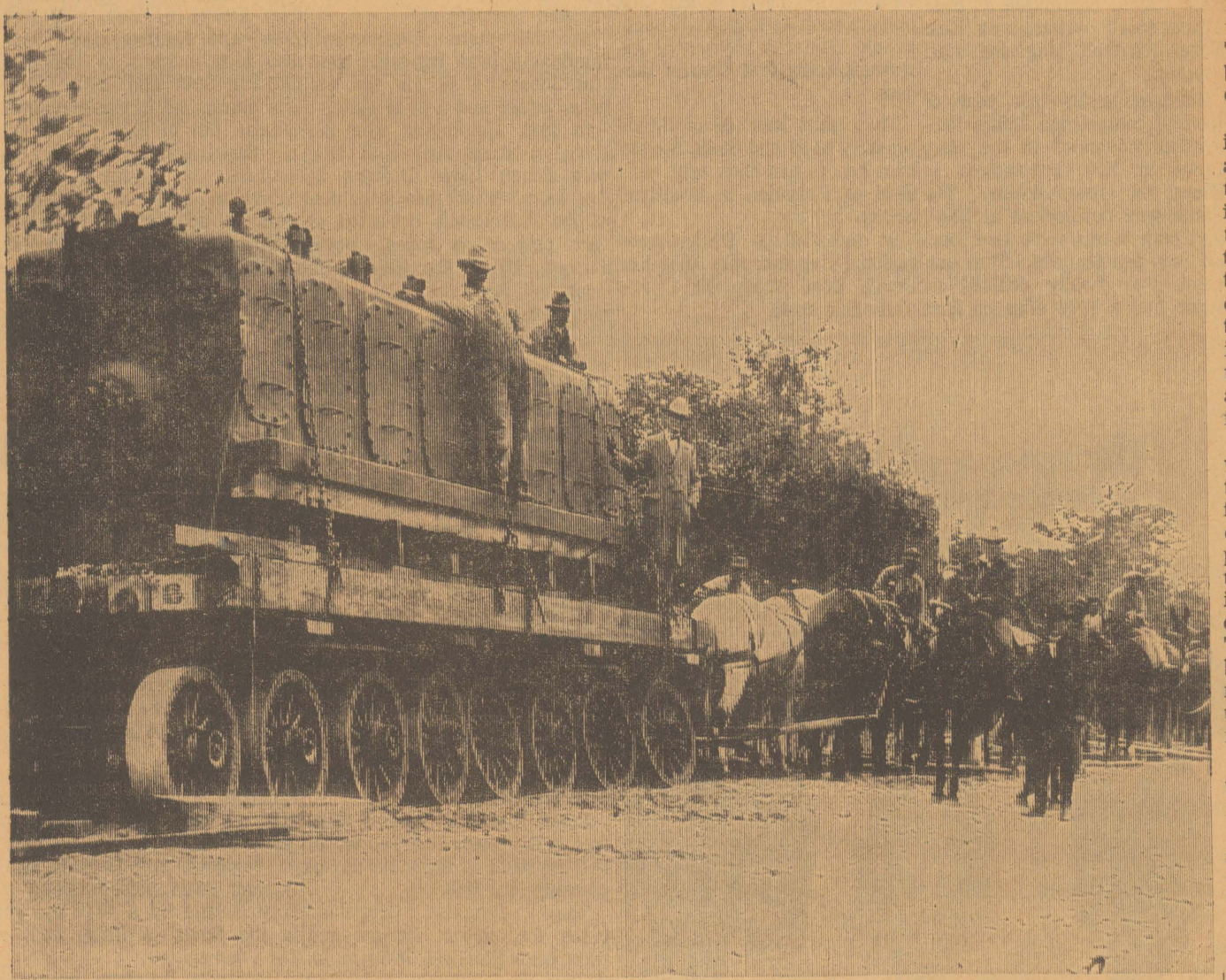
THIS IS THE WAY it once was done. A forerunner of the Lufkin-built trailer vans and floats was this 16-wheel wagon built by Martin Wagon Co. Here a large piece of machinery was being hauled to the Gulf Pump Station during its construction north of Lufkin. Picture was made in 1925.
