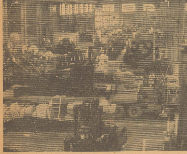
ASSEMBLY building where component parts of pump units are assembled and shipped to world markets.
