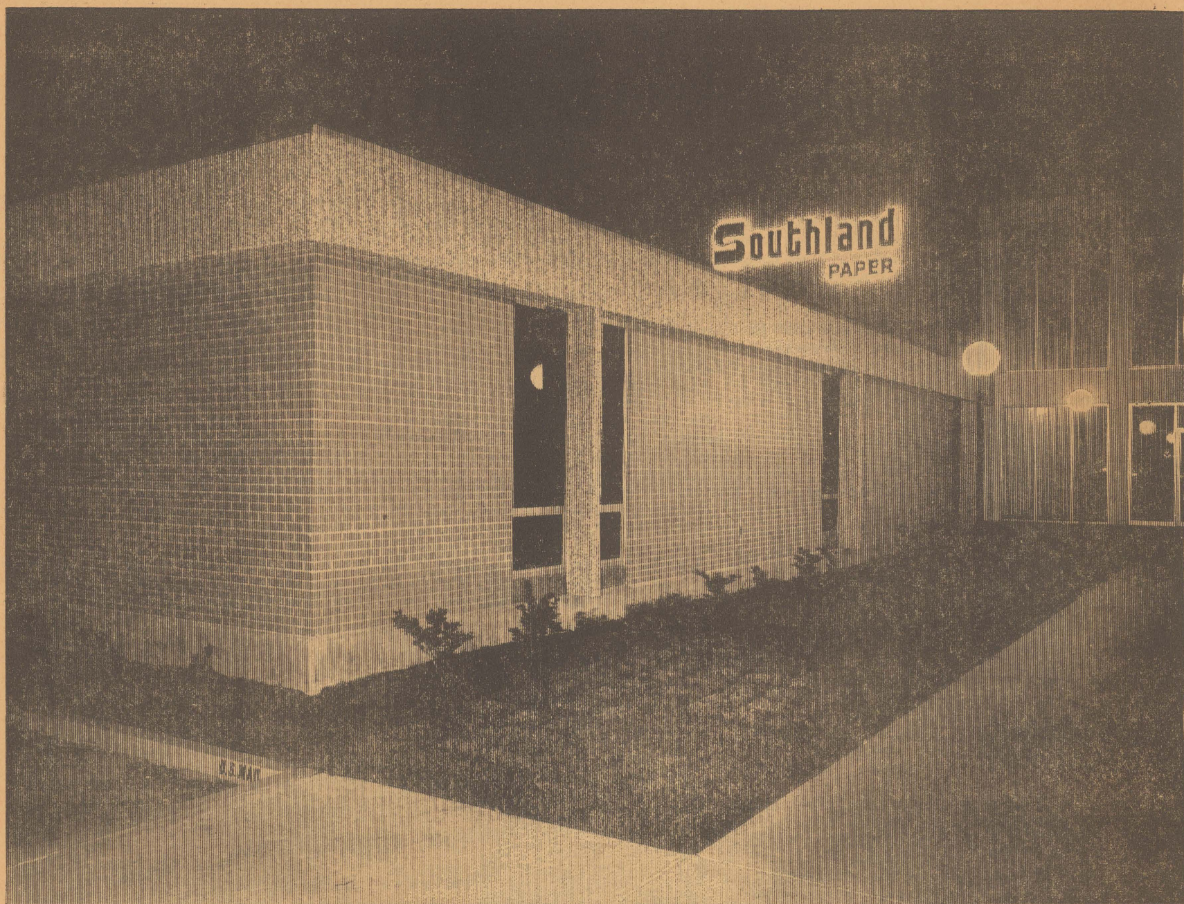
NEW BUILDING HOUSES SOUTHLAND'S FOREST OPERATIONS ... addition to company's headquarters building
