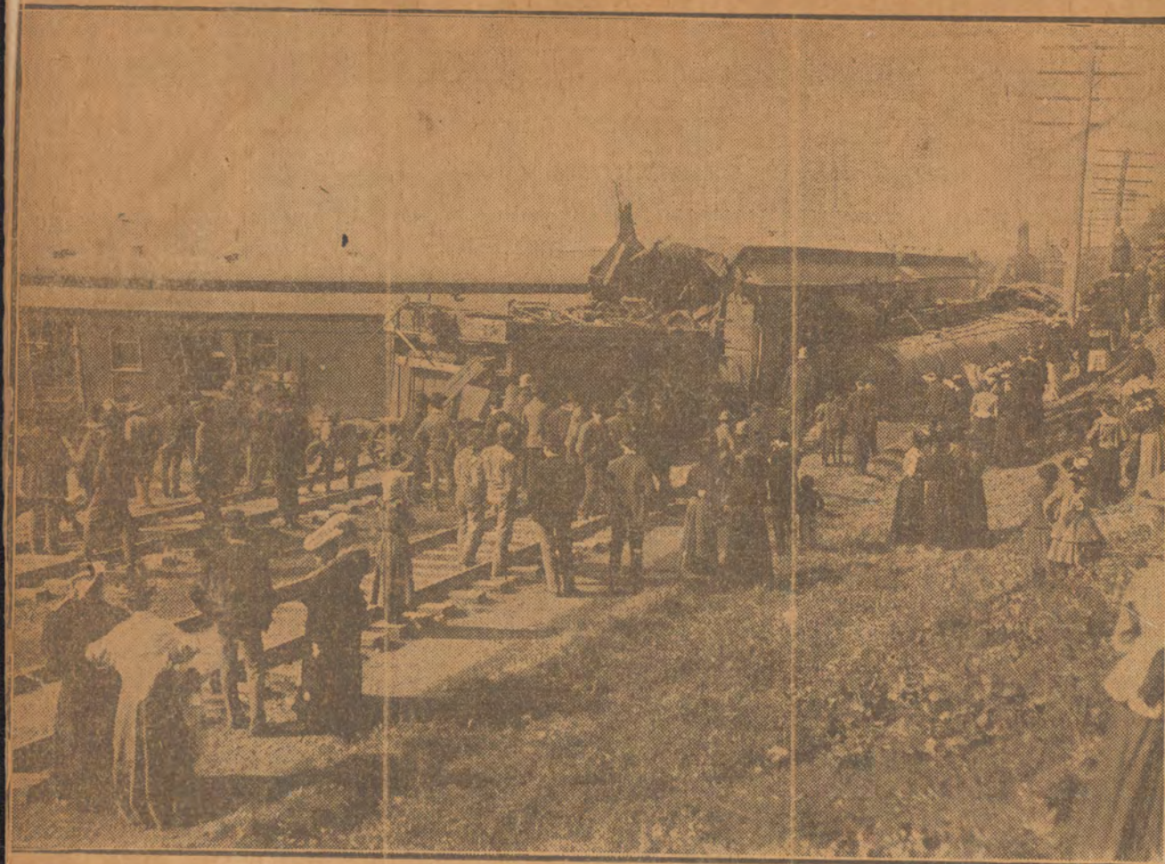
When the Engine and Baggage Cars Left the Track They Were Piled Up on the Embankment at the Side, the Locomotive Turning Over and Half Burying Itself in the Soft Earth.
