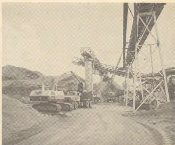
New overhead chip conveyors under construction in chip yard. Excavation at left is for new chip reclaim tunnel.
