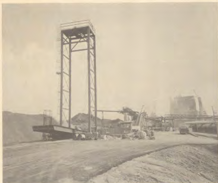
New chip truck dump platform and lift tower at north end of mill [looking south].
