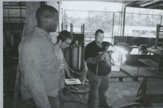
E. Phipps, J. Mewborn watch C. Carrell strikes up a cutting torch to pop some holes into the trailer ramps.
