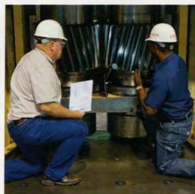
Lufkin Gear Repair .....
