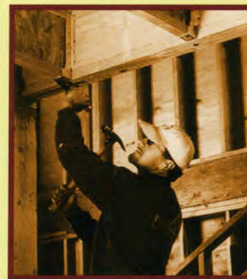
Workman installing Rosboro Lumber's Big Beam product.
