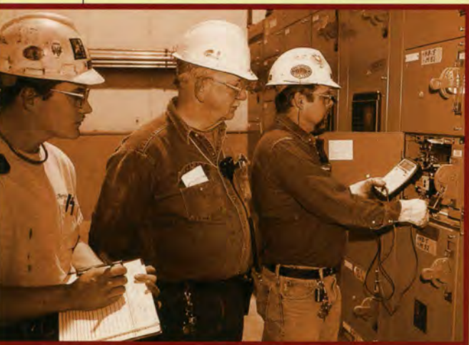
Maintenance Technician Scott Loe observes Walt Doege, maintenance technician, and Robbie Miller, electrical lead, demonstrate proper lock out procedures for testing electrical equipment at Hope Particleboard Operation.
