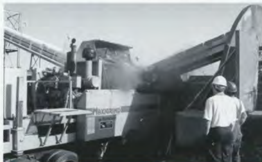
Gypsum Grinder at Fletcher, OK.
