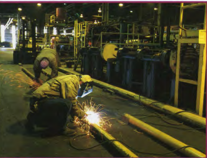
Johnny Perry, millwright-A, and R.L. Wright, millwright-A and welding specialist, are among the employees that recorded 738,527 man-hours worked with no lost time accidents.
