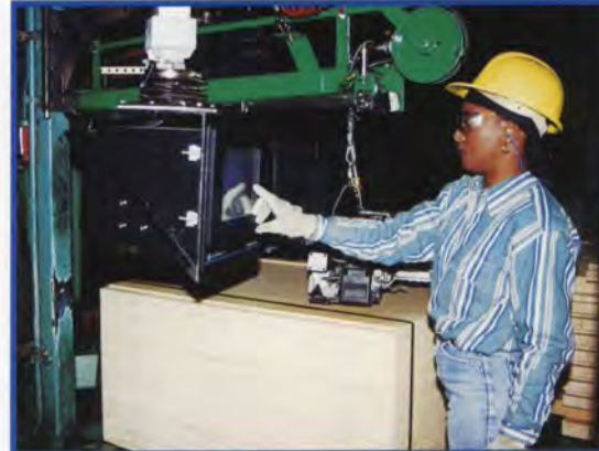
Deborah Benton utilizes the newly installed panelview touchscreen controller at the strapper at Diboll Particleboard Operation.
