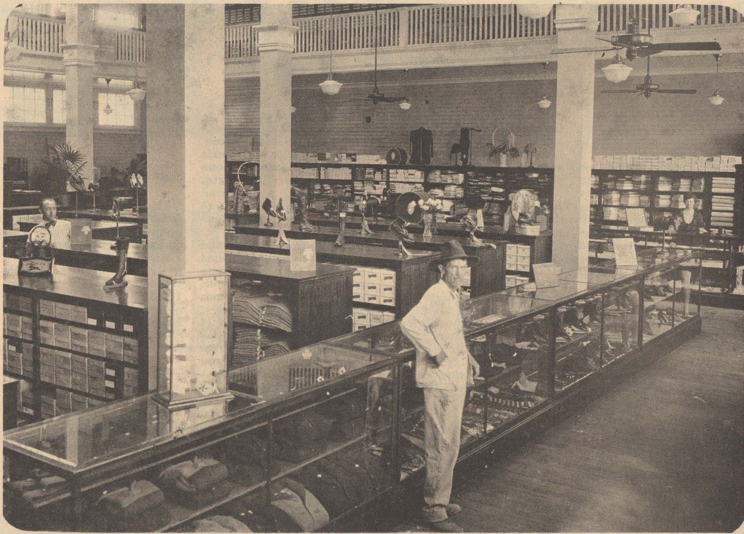
Company commissary was a complete general store for employees
