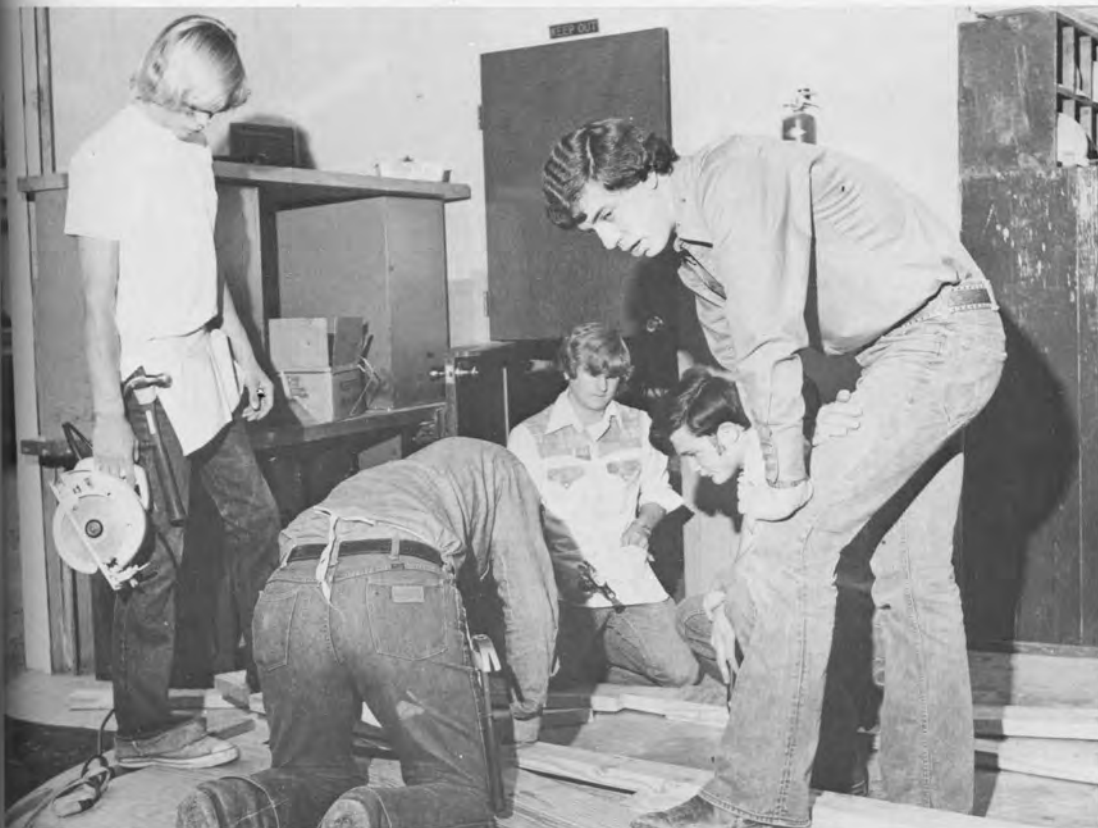
V. I. C. A. Club Boys Work on Housing Project
