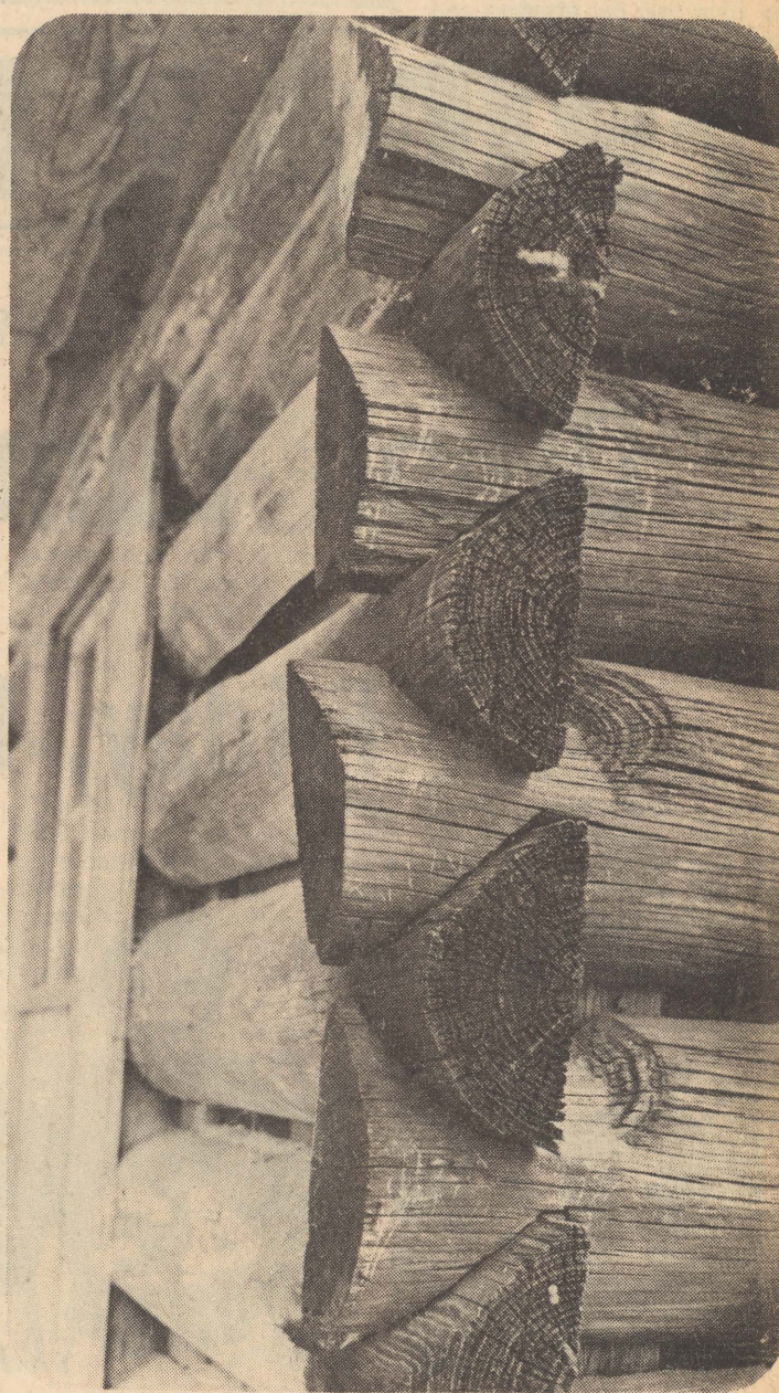
Logs are notched neatly into place at corners
