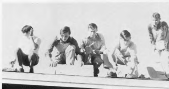
Boys work on house.
