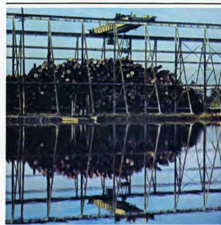
The modern tree-length log processing yard at Diboll directs log inventory to several locations, assuring maximum utilization.
