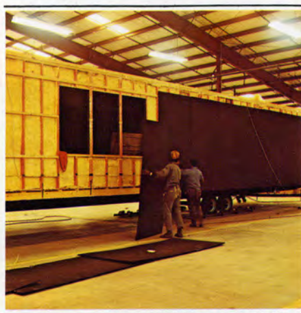
Many Temple products, including lumber and fiberboard, are used in the construction of mobile homes.
